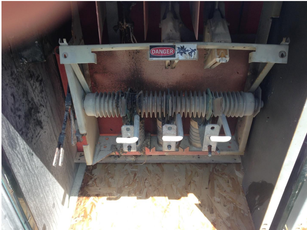
Figure 5.3-42: Example of a Failed Switchgear
