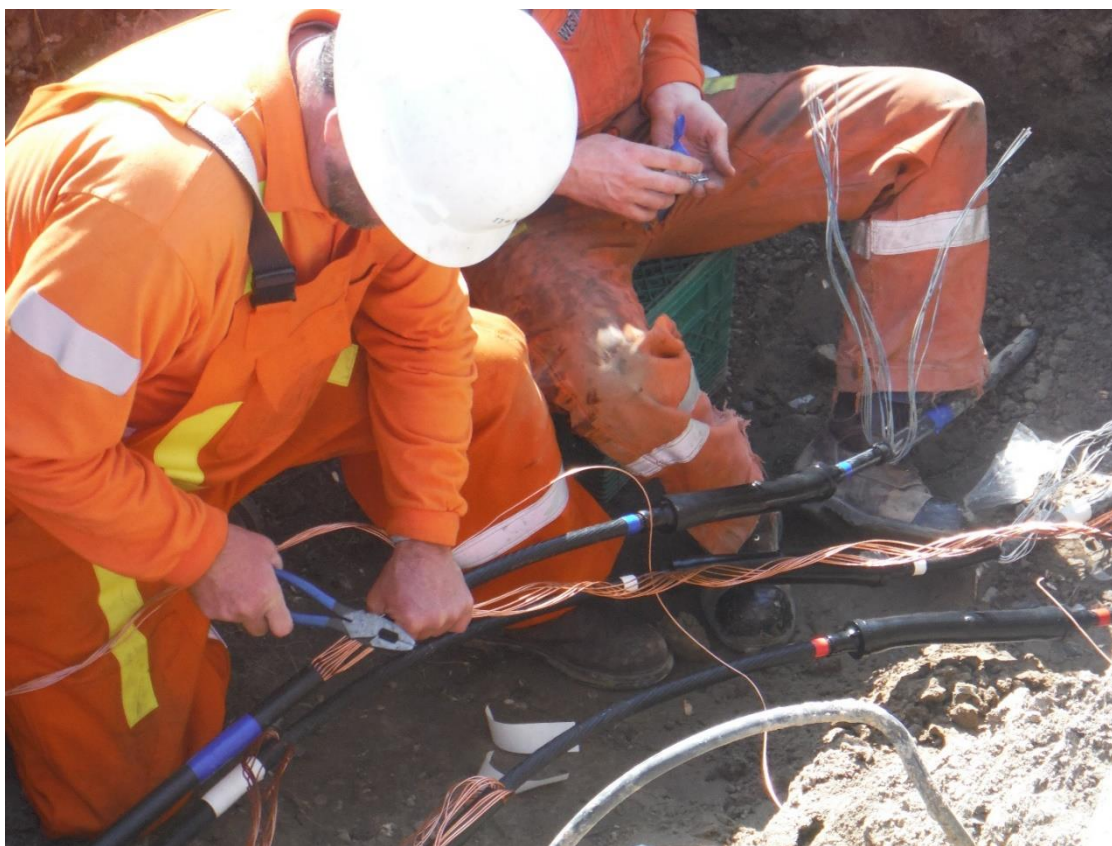
Figure 5.3-36: Work Crew Completing a Cable Splice
