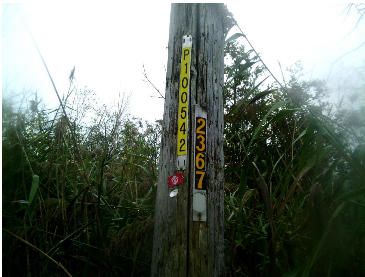
Figure 5.3-35: Example of Pole with Signs of Deterioration (2)
