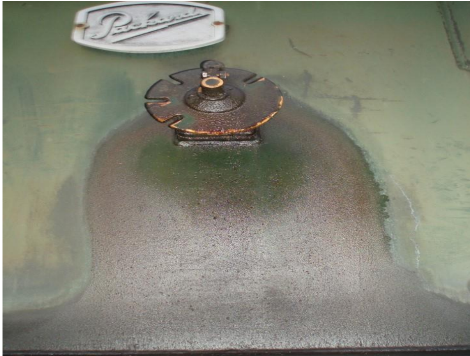
Figure 5.3-40: Example of Leaking Oil Valve in Pad-Mounted Transformer
