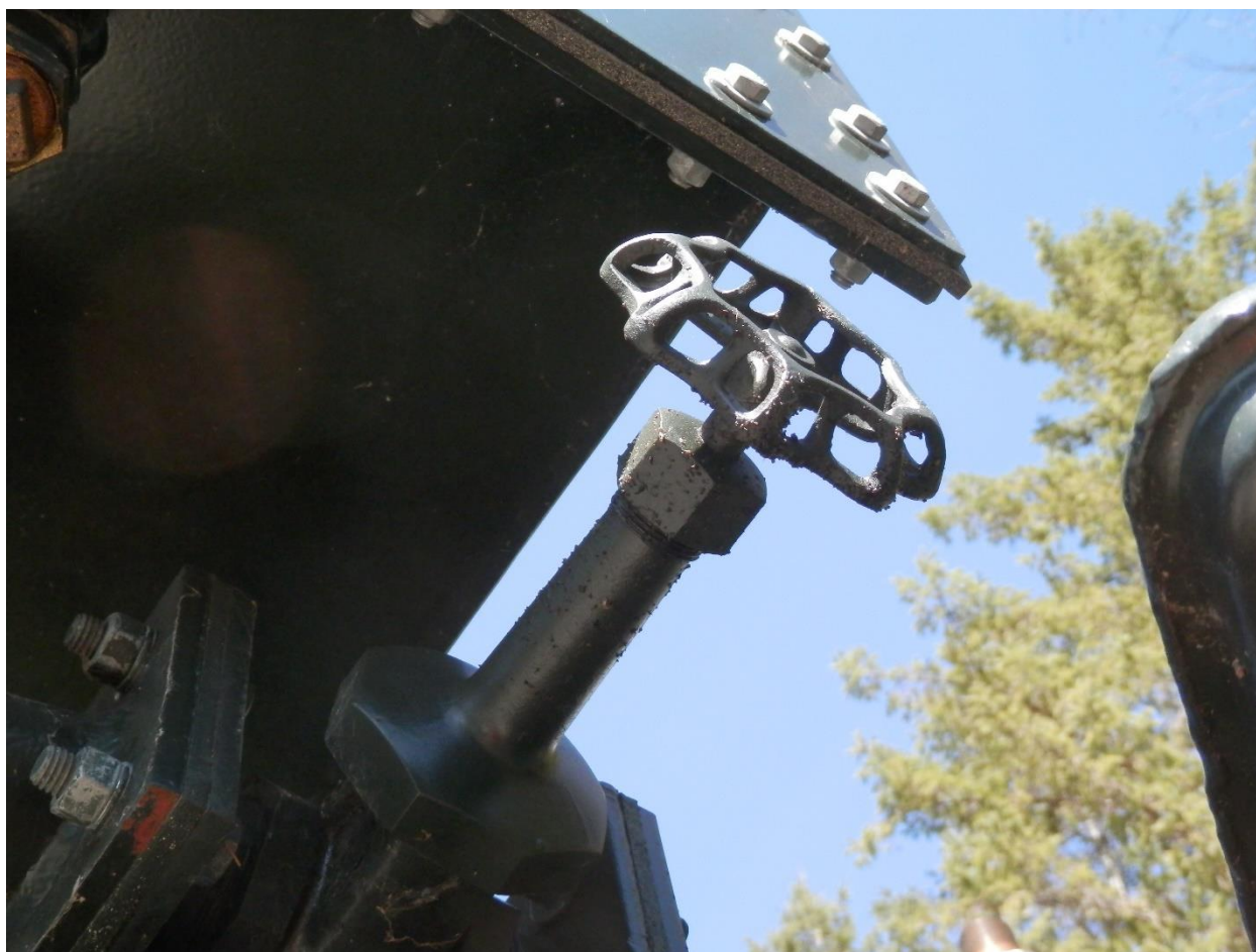
Figure 5.3-43: Example of Power Transformer Conservator Valve with Signs of Leaking
