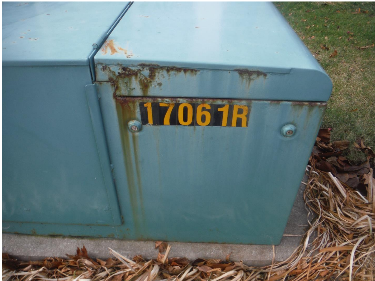
Figure 5.3-38: Example of Pad Mounted TX with Signs of Deterioration (1)
