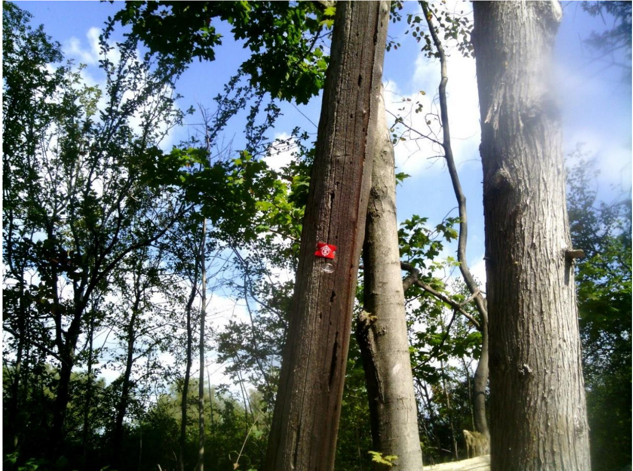
Figure 5.3-34: Example of a Pole with Signs of Deterioration (1)
