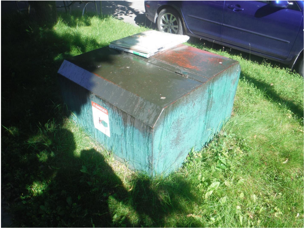
Figure 5.3-39: Example of Pad Mounted TX with Signs of Deterioration (2)
